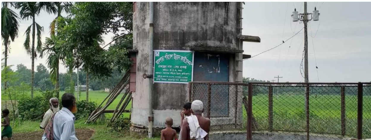
Figure 25: Established deep-tubewell for round the year irrigation and household water supply
